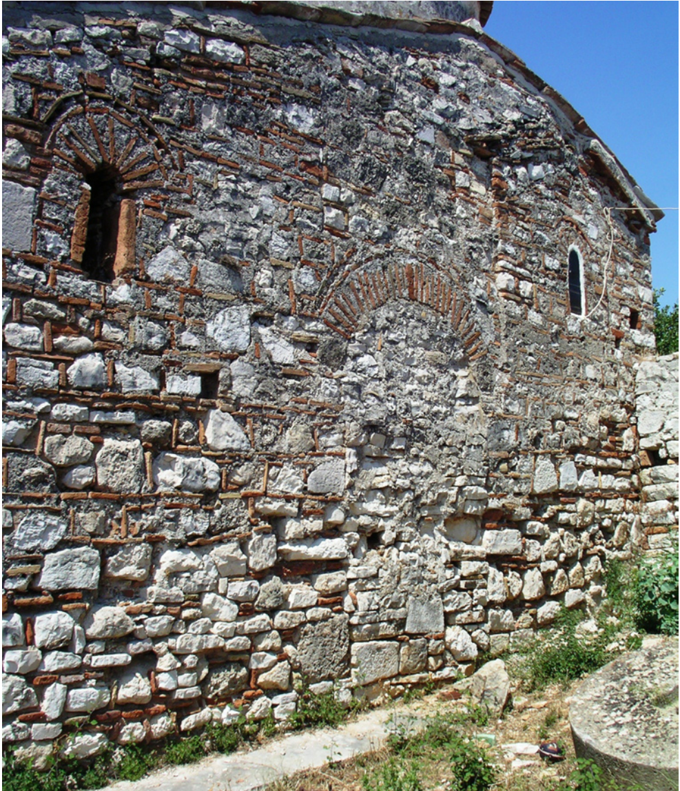
Fig. 75. Koronissia, Panagia Monastery, katholikon. View of the S façade from S.
